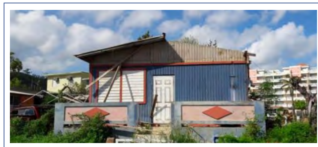
Construction materials common in Puerto Rico, such as corrugated metal roofs, must be accounted for in model databases for accurate loss estimation. Photo: Strategic Alliance for Risk Reduction (FEMA contractor)
